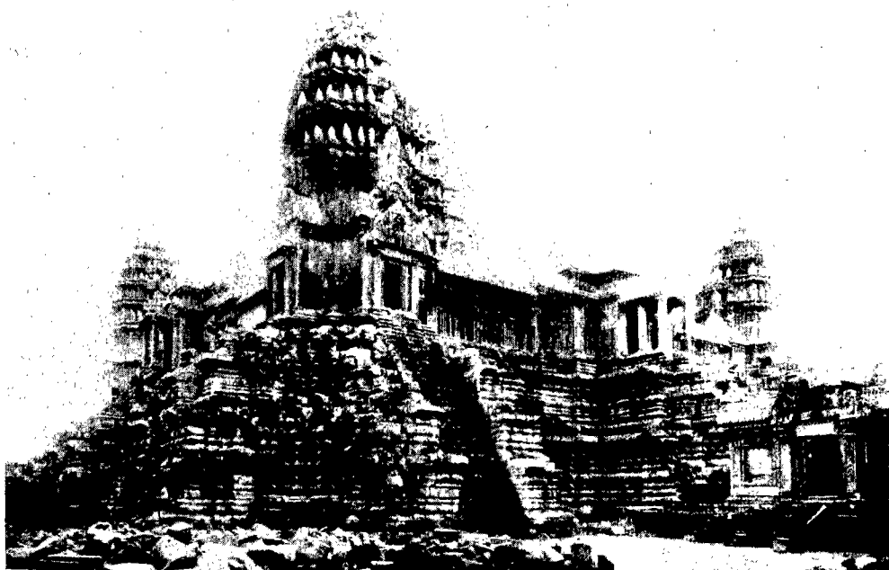
Angkor-Vat, a general view, third story in Angkor, Kingdom of Cambodia or Khmer, in Indo-China. The third tier of galleries rests on an enormous square basement, each face of it being 82 yards long. Twelve monumental staircases lead to these galleries. At each corner rises a tower. From the ground up to the top of these towers all has been drawn, engraved and pounced by masters
