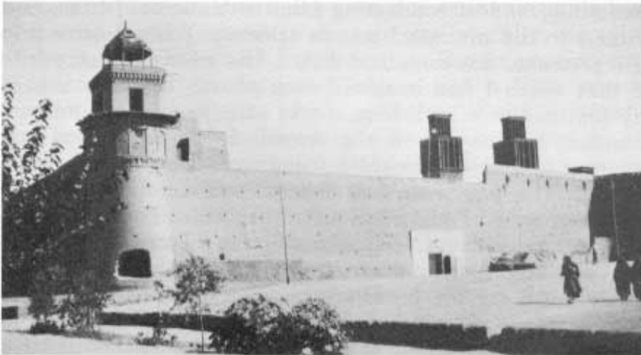
VIEWS OF THE FORT OF NĀRĪN, YAZD
