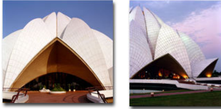
Figure 3.73: (l-r) Views of the Entry Points to the Temple showing the red sandstone Walkway/Entry flooring, curved Balustrade and white marble shells Source: http://en.wikipedia.org/wiki/Lotus_Temple
