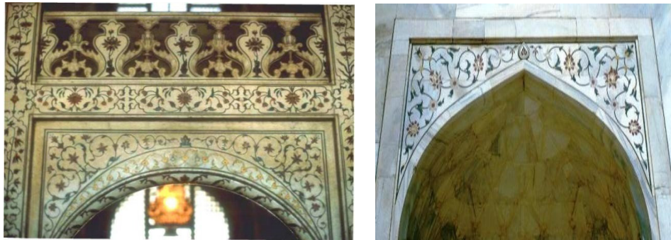
Figure 3.66: (l-r) Arch of Jali showing delicate inlays and Spandrel details over Main Iwan Source: http://en.wikipedia.org/wiki/File:Taj_Decorations.jpg http://en.wikipedia.org/wiki/Taj_Mahal
