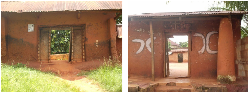
Figure 3.27: (l-r) Entrance gate into the Palace of HRH Chief J.N.Ofomata ‘Obu of Nanka’ and entrance gate into the Palace of Obi Onyiuke Nimo both in Anambra State. Source: Author’s field photos, 2008
