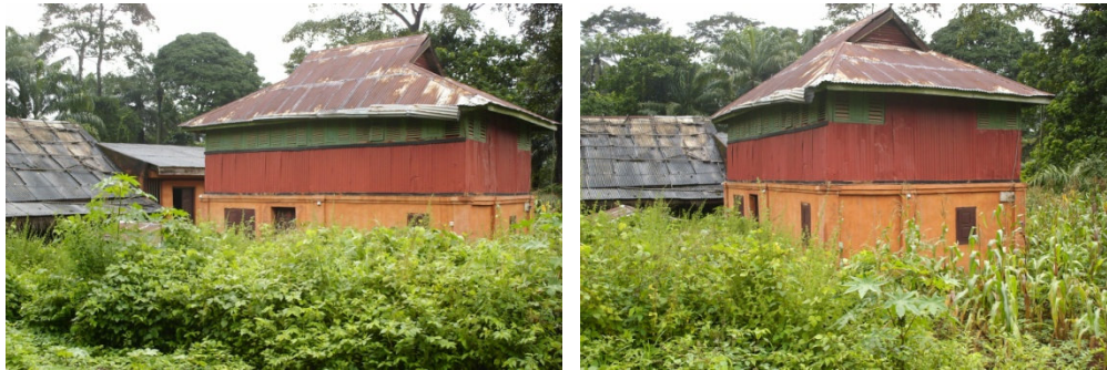
Figure 3.84: Chief Nwodo's Storey Building within the compound overgrown with weeds. The upper level is covered with corrugated steel sheets (red) and timber jalousie windows (green) Source: Author's Field Photos, 2009.
