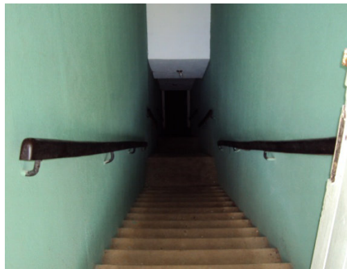
Figure 3.83: Top (l-r), Rear view of the Biafran Government House, covered walkway from the Courtyard leading to the entrance of the Bunker; Bottom, Entrance of the Bunker Source: Author's Field Photos, 2011
