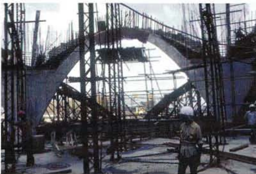
View showing newly concreted main arches
