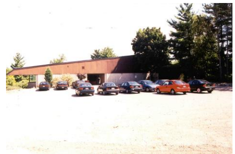
Fig. 3: Back view of National Bahá'í Centre looking east.
