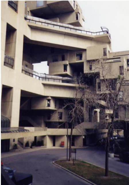
Fig. 1: Habitat '67 designed by Moshe Safdie for Expo '67.
