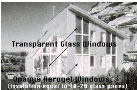
Fig. 9: Test site comparing aerogel filled units to normal glazing units.
