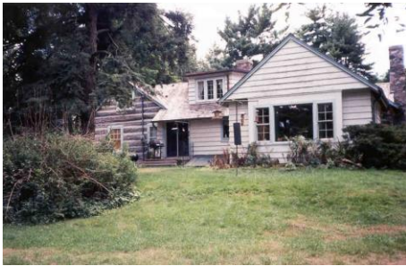
Fig. 9: Back view of heritage building, circa 1950.
